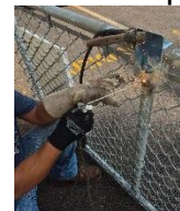
Welding Fence Repair
