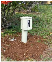
New Breaker for Lalo Heat Pump and Charging Station for Maintenance Carts.
