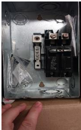
New Breaker for Lalo Heat Pump and Charging Station for Maintenance Carts.
