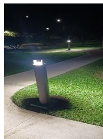
Completed path light upgrade near Building 7. They are sturdier and more weatherproof
