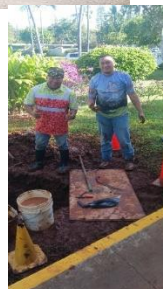
Fixed main line water leak near the KEE Pavilion.
